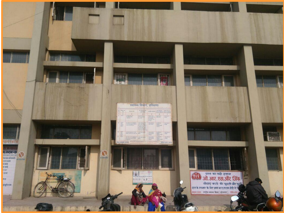
Civil Hospital, Jhajjar
